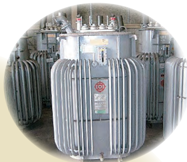
■ PCB-containing transformer
