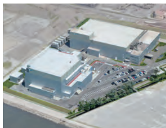
■ Hokkaido PCB Treatment Facility
