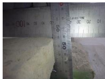
切削深さ確認
